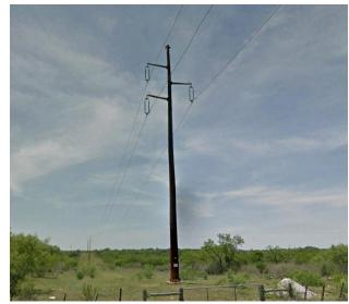
AEP Texas representatives plan to use single pole, weathered steel structures.
